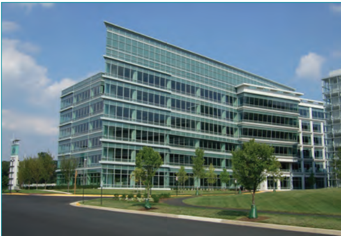
Dulles Station East delivered 180,000 square feet of speculative office space in January 2008.
