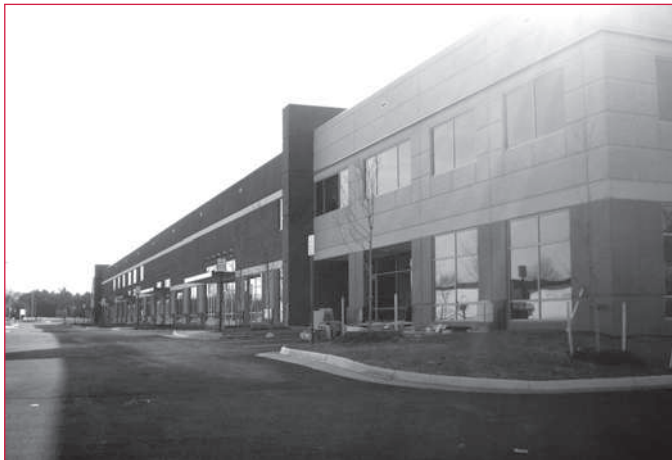
Towerview Commerce Center in Dulles delivered 57,011 square feet of industrial condo space in December 2007.
